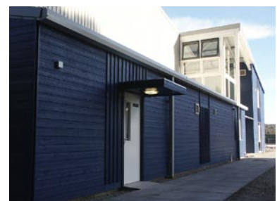
This Leisure Centre in Lochinver, Sutherland was pressure tested to ensure that the designed energy efficiency measures would lead to the anticipated energy savings for the Client. Design: Gaia Architects. Source: C. Morgan.
