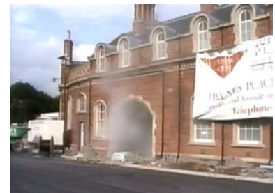
... which are then immediately visible! Source: HRS Services Ltd. www.air-tightness.co.uk
