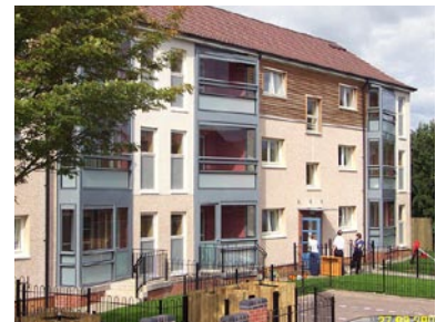
This refurbishment of 1950s tenements in Fife by John Gilbert Architects included airtightness measures as part of overall energy efficiency improvements. Source: J. Gilbert.
