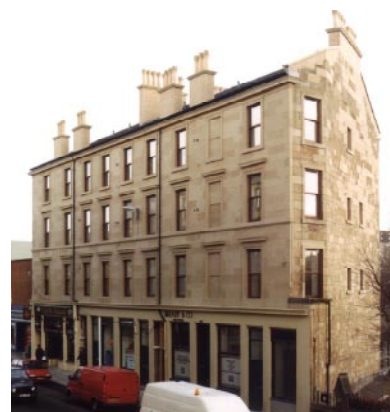
This Glasgow tenement was refurbished using a variety of energy efficiency measures including airtightness. Source: J. Gilbert.
