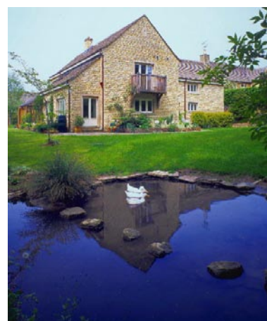
In Canada, ordinary dwellings are routinely built to an airtightness of around 3 m 3 /hr/m 2 at 50 Pa (BRE IP 1/00). Even in the UK, the house above, by David Olivier of Energy Advisory Associates achieved a monitored airtightness of 3.3 m 3 /m 2 hr @ 50 Pa, before remedial works. Source: D. Olivier.
