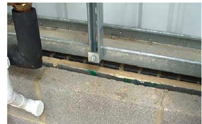
Gaps between blockwork and steel, above, and uncapped cavity wall at join with composite panels, below. Source: P; Jennings
