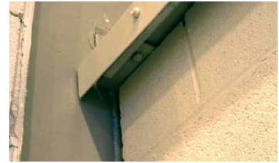
Gaps between blockwork and steel, above, and uncapped cavity wall at join with composite panels, below. Source: P; Jennings
