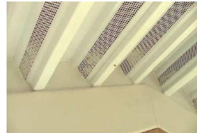
Missing profile fillers, top, and perforated liner sheets which extend through into the cavity at the verge, above. Two examples of gaps around windows, below and bottom, two examples of gaps around services penetrations within the building. Source: P. Jennings.
