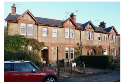
Older properties tend to suffer in particular from draughty suspended timber floors and gaps within, and around windows and doors. Source: C. Morgan.
