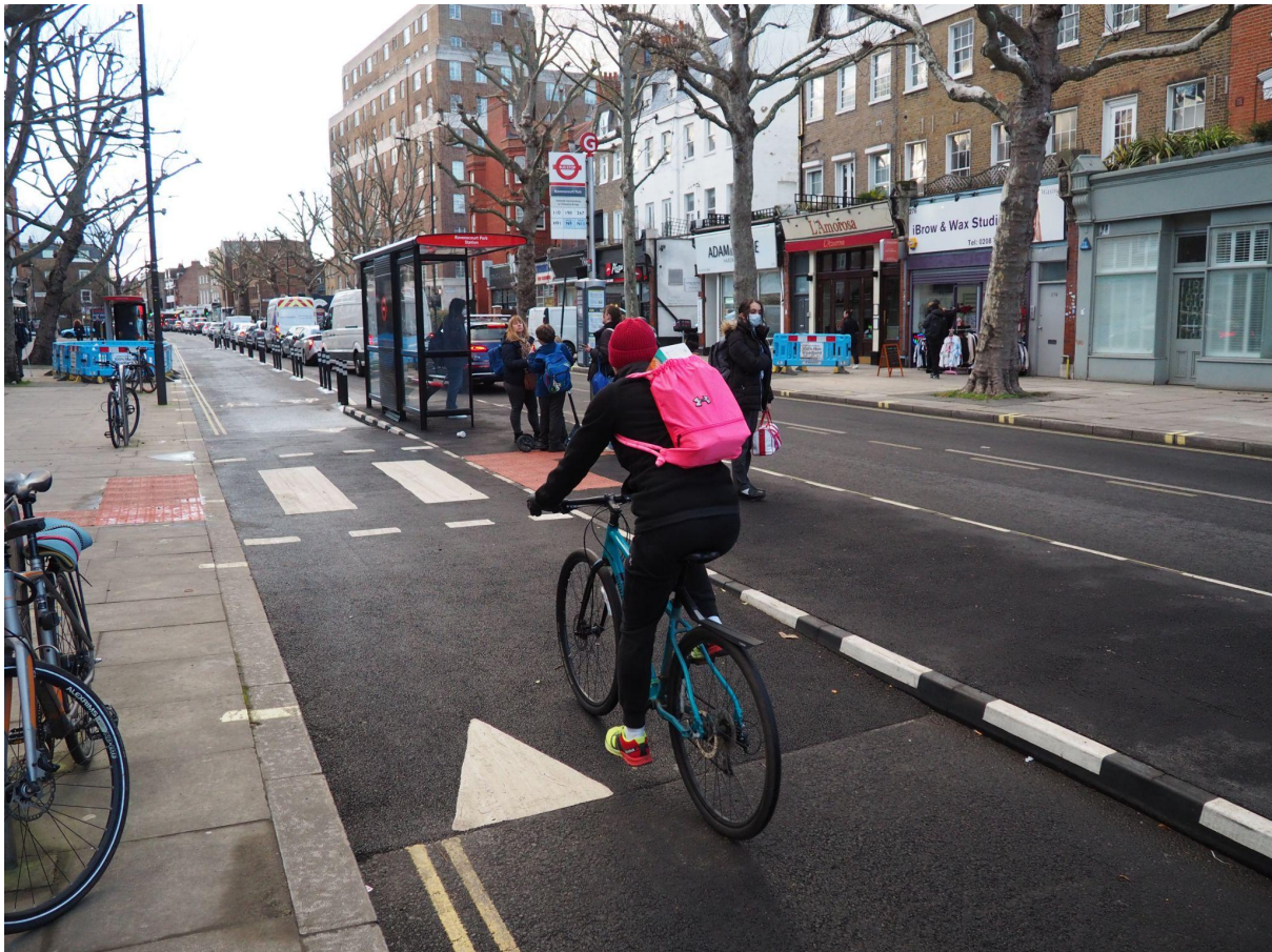
A bus stop bypass in Hammersmith, West London, showing some of the elements recommended by the RNIB (contrasting tactile paving to show a crossing point, zebra markings, detectable upstands and kerb separation delineating the pavement, lane and bus stop island, and a ramp for slowing of the cycleway). Photo: Leo Murray
